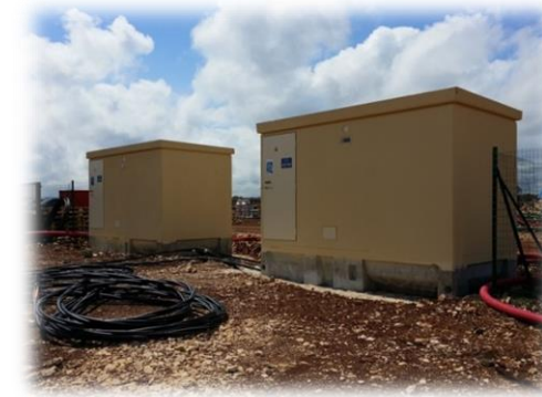
Pose de postes HTA
